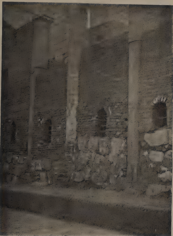
FIG. 121.—The White Monastery : Walled-in columns of nave. (Photo. by J. G. M.)
